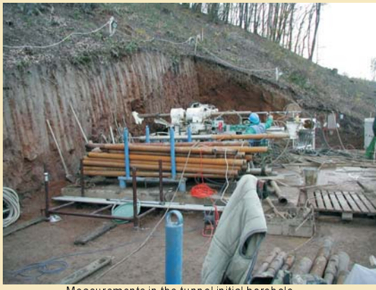
Measurements in the tunnel initial borehole
