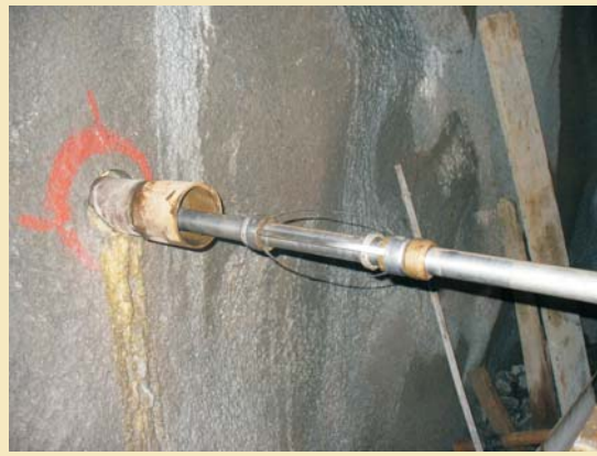
Probe insertion of horizontal drilling
