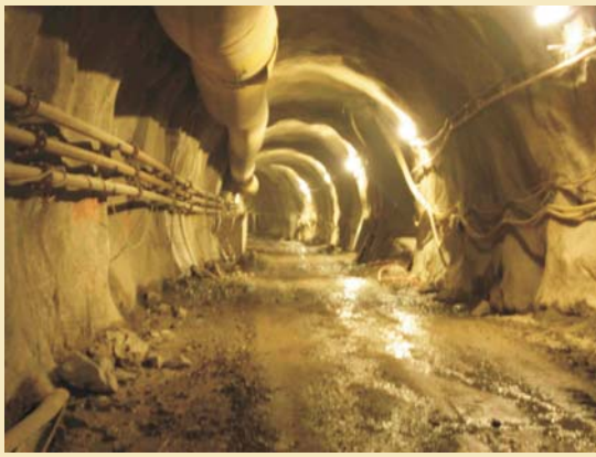
Inside the tunnel
