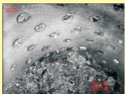
Sediment accumulation in plastic screen pipe
